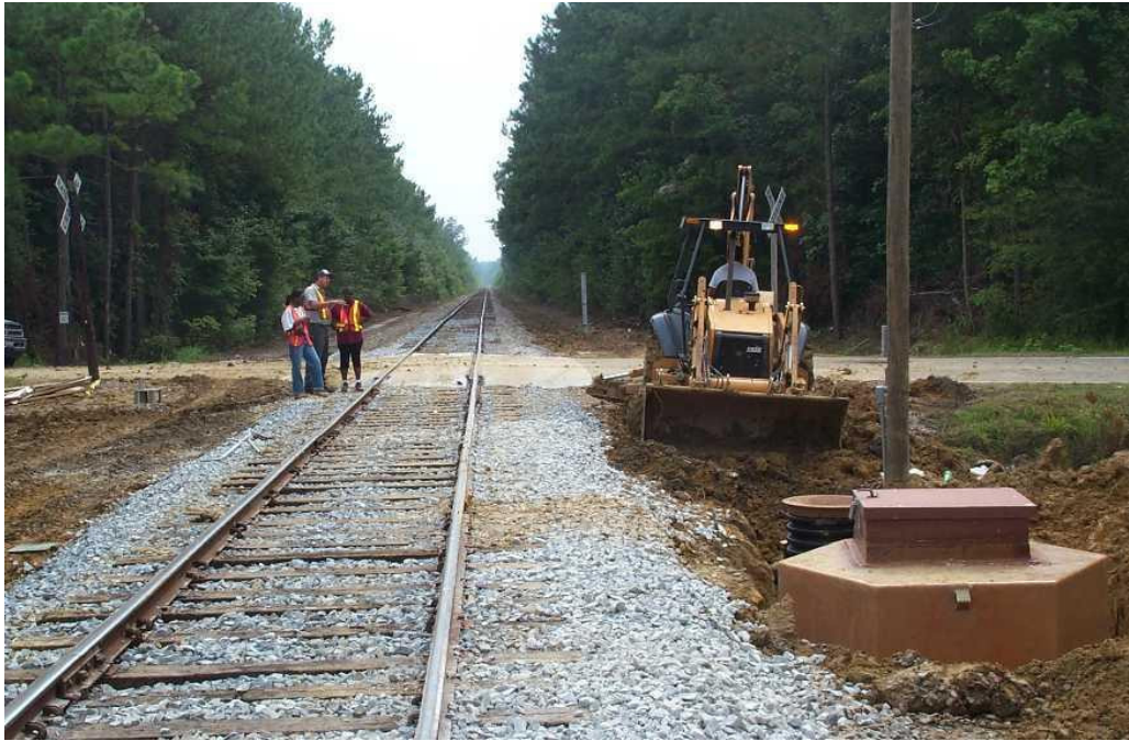
Figure 3.3 – Vault filling
