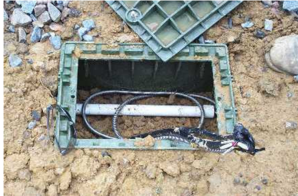
Figure 3.2 – Installed Magnetometer
